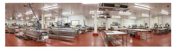
A high-strength industrial floor coating over all concrete slabs in the food processing area prevents food particles from absorbing into the concrete slab and minimizes the risk of bacterial growth. (Photo courtesy of A M King.)
