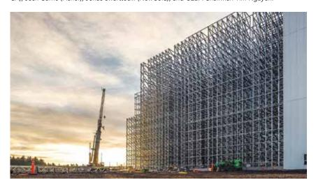
The NewCold Tacoma state-of-the-art freezer is a joint design effort by Netherlands-based NewCold Advanced Cold Logistics and the design/build firm Fisher Construction Group of Burlington, Washington. It is one of the largest cold storage facilities in the United States, with Phase 1 containing approximately 25 million cubic feet of storage capacity an 103,000 pallet positions. ((Photo courtesy of NewCold.)
