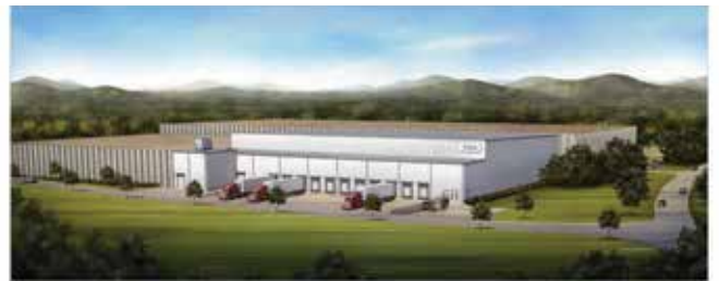
Winchester Cold Storage, Winchester, Virginia
