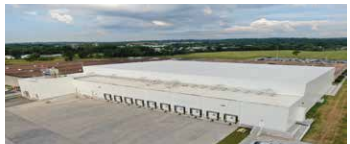
Winchester Cold Storage, Winchester, Virginia
