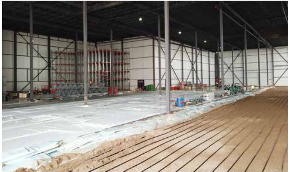
In the background, progress is shown of an expedited zone that was needed while floors were still being established (in the foreground) and racking installed. (Photo courtesy of Coldbox.)
