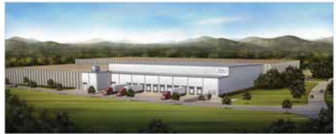
Winchester Cold Storage, Winchester, Virginia
