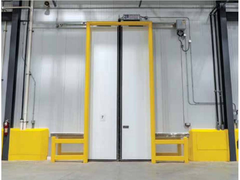
The bi-parting doors were supplied by ASI Doors. (Photo courtesy of Dick Cold Storage.)
