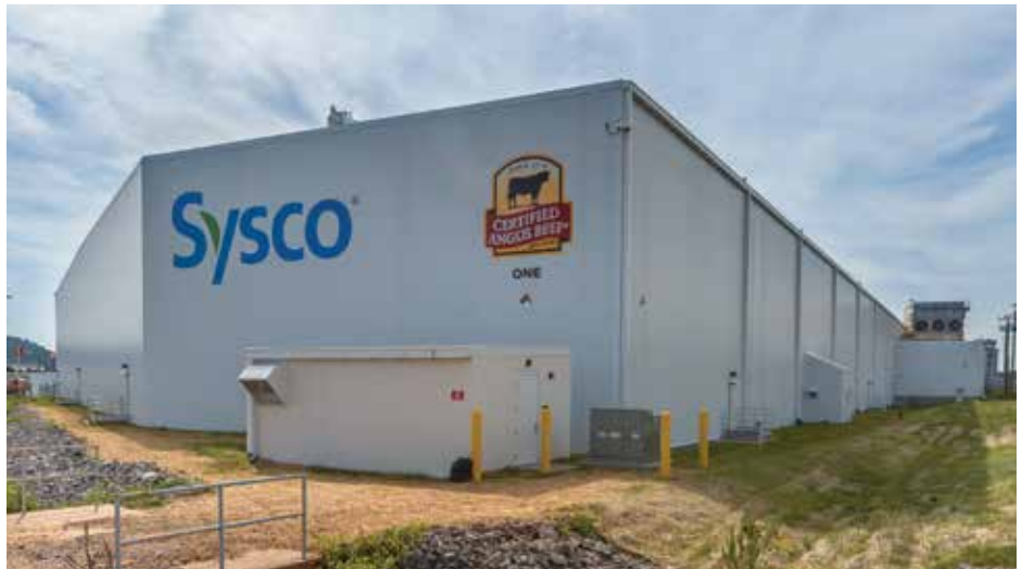
Sysco Nashville looked to Williams Company to build back even better after a tornado ripped through the facility. (Photo courtesy of Williams Company.)
