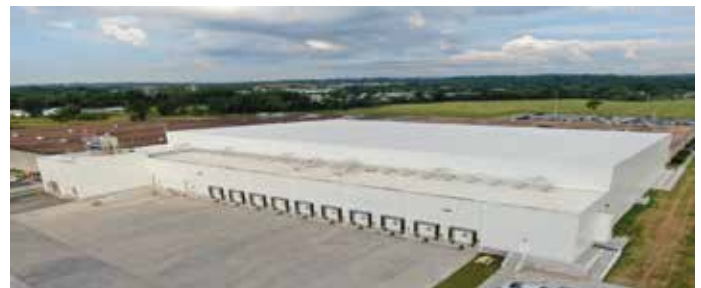
Winchester Cold Storage, Winchester, Virginia
