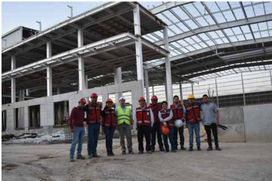
SRT was hired to design/build a distribution center in Mexico City, Mexico, for Mexideli, that would unite the company's operations in a single facility. (Photo courtesy of SRT.)
