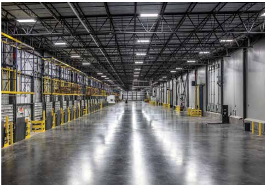
ARCO Design/Build created a cold storage facility for MTC Logistics capable of processing a million pounds each day. (Photo courtesy of ARCO Design/Build.)
