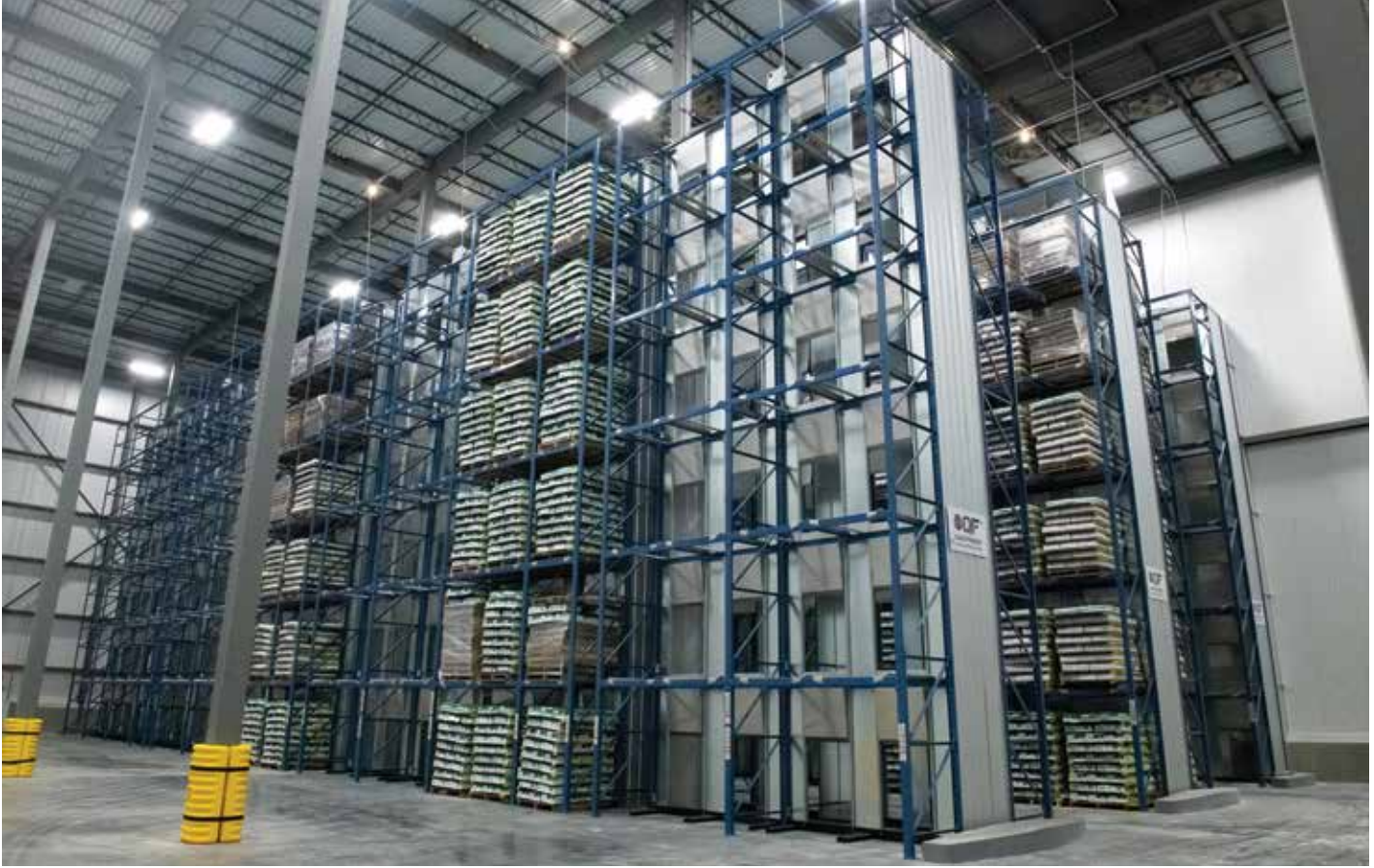
To create as much storage space as possible on the allotted site footprint, innovative racking solutions were implemented. (Photo courtesy of ARCO Design/Build.)
