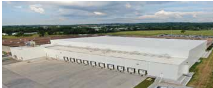
Winchester Cold Storage, Winchester, Virginia
