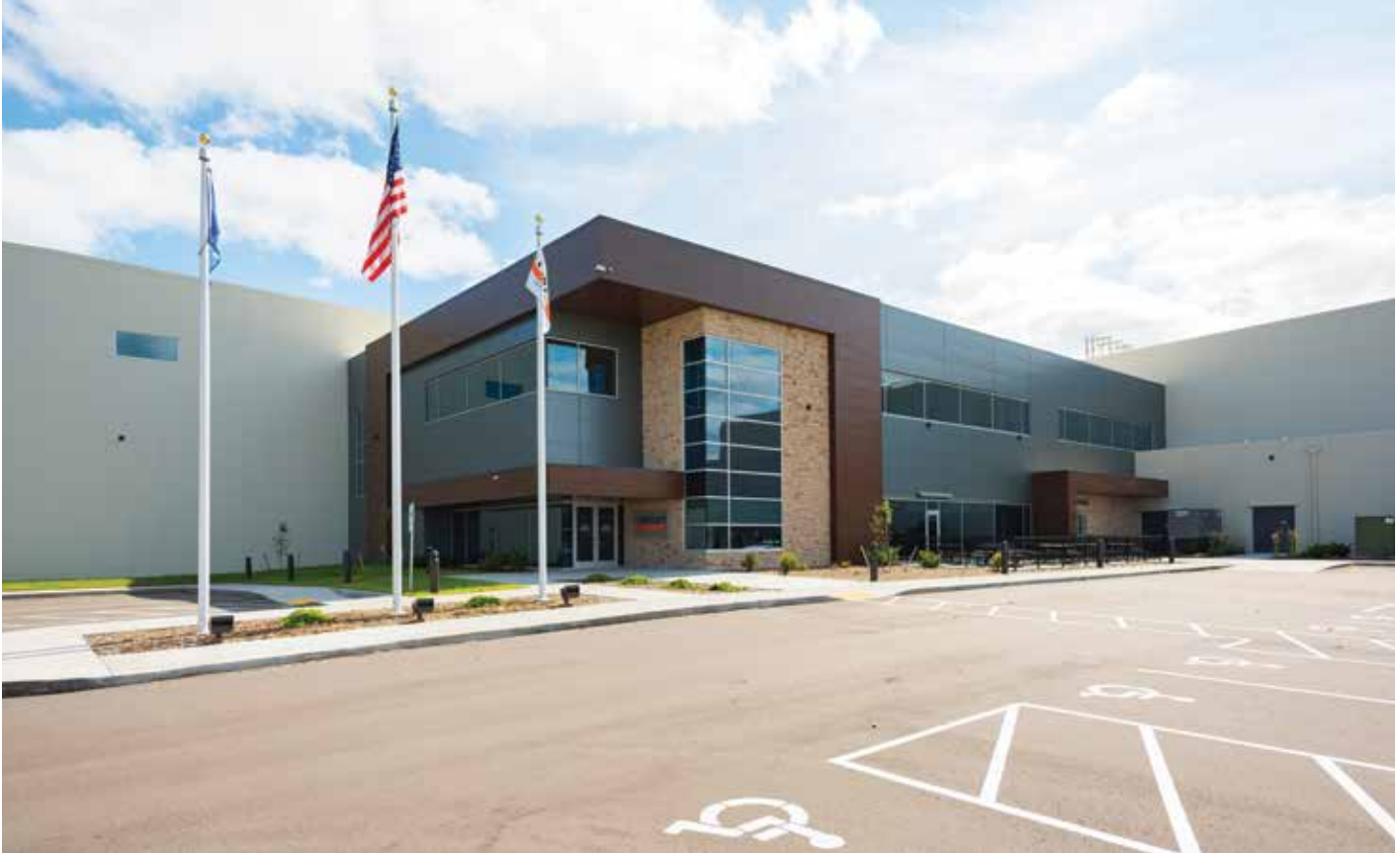
The 242,706-square-foot facility was designed for Performance Food Group by ESI for multiple uses with its primary purpose to distribute food to the local region. (Photo credit Curtis Waltz, Aerialscapes. Photo courtesy of ESI Group USA.)
