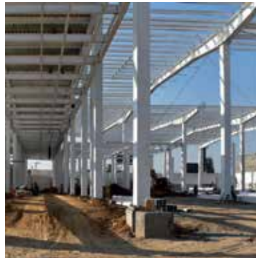
Civil works and structure
