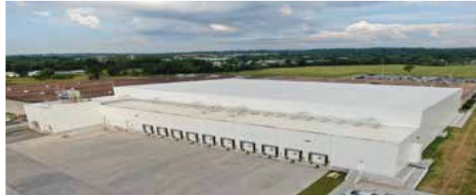
Winchester Cold Storage, Winchester, Virginia
