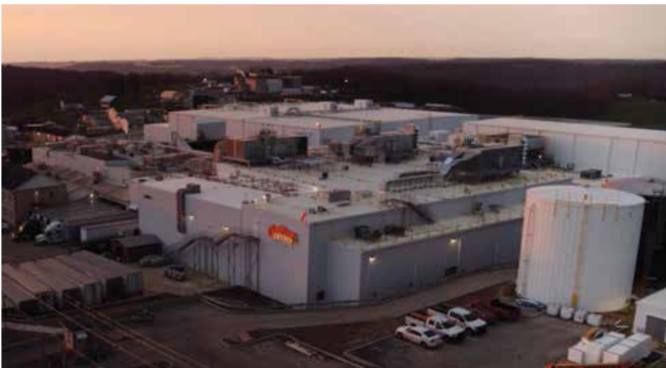
(Photo courtesy of Primus Builders, Inc.)
