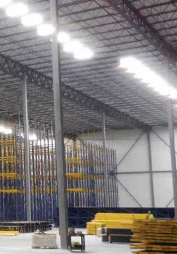
A fully automated mobile racking system in a -10F freezer space. The mobile rack system moves on steel rails embedded into the floor system and is designed for one forklift aisle in every column bay. (Photo courtesy of ARCO Design/Build.)
