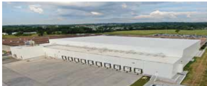
Winchester Cold Storage, Winchester, Virginia
