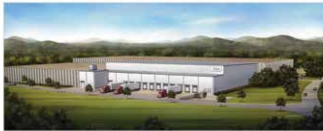
Winchester Cold Storage, Winchester, Virginia
