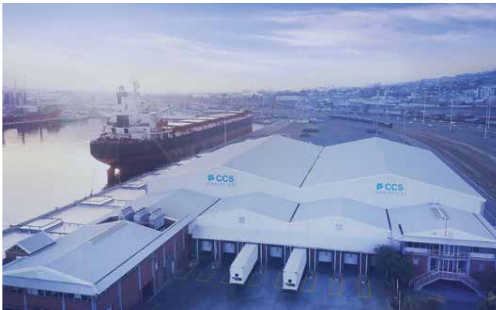
CCS Logistics at Duncan Dock, Capetown, South Africa. (Photo courtesy of CCS Logistics.)
