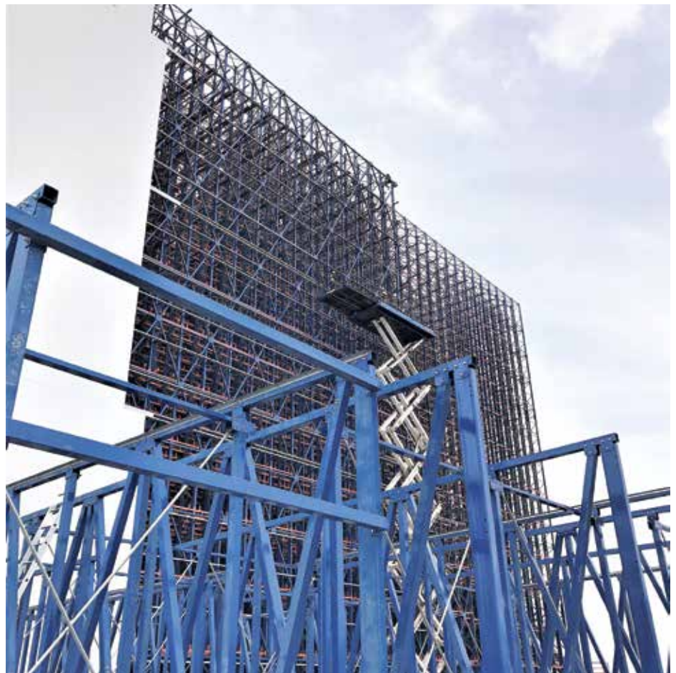
An ASRS shuttle-type facility with 80,000 pallet freezer. (Photo courtesy of Coldbox Builders.)
