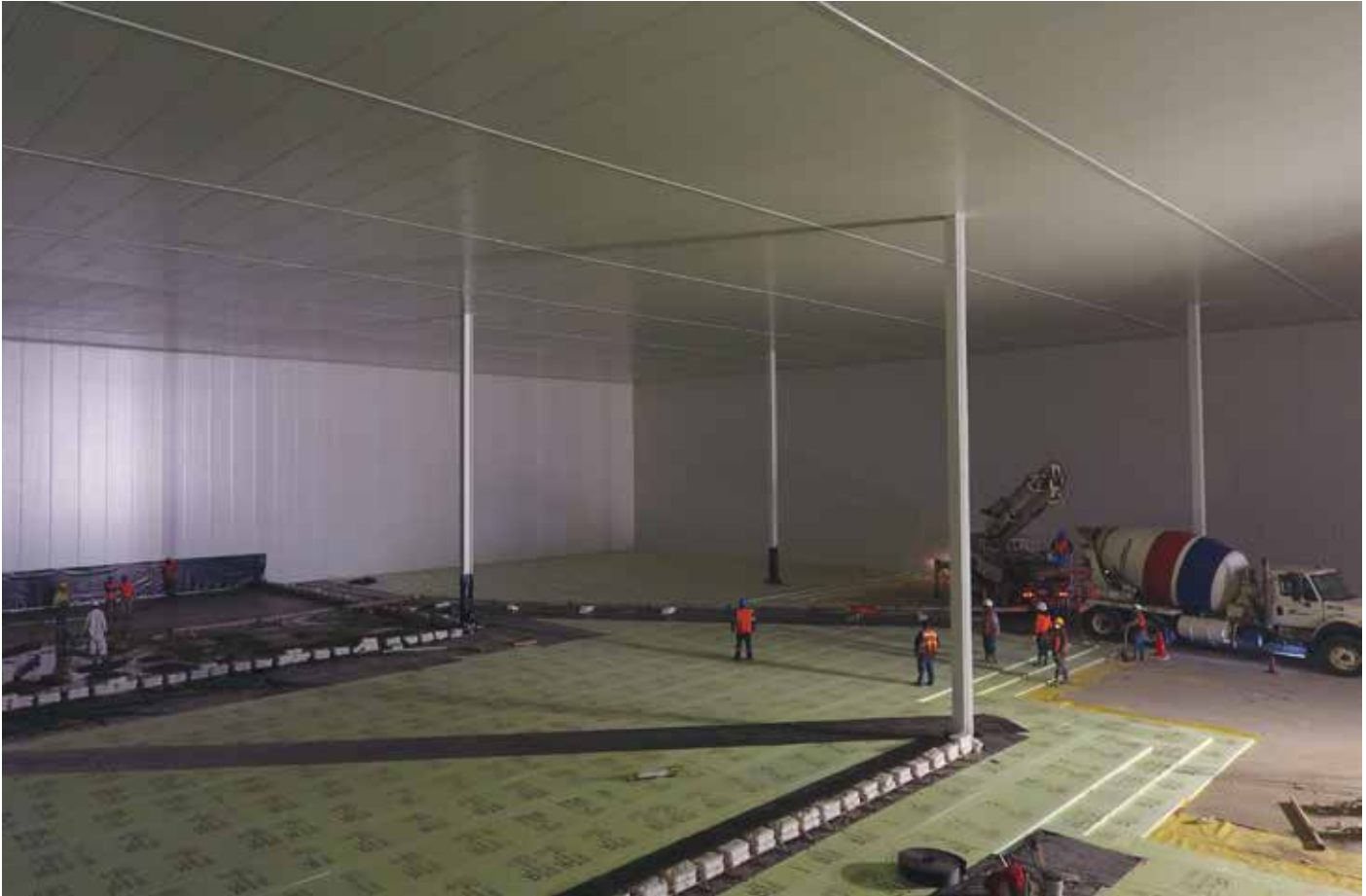
A 13,000-square-meter cold storage warehouse capable of reaching -20 °C built in 2018 by Infrisa in Tijuana, Baja California, Mexico. (Photo courtesy of Infrisa.)
