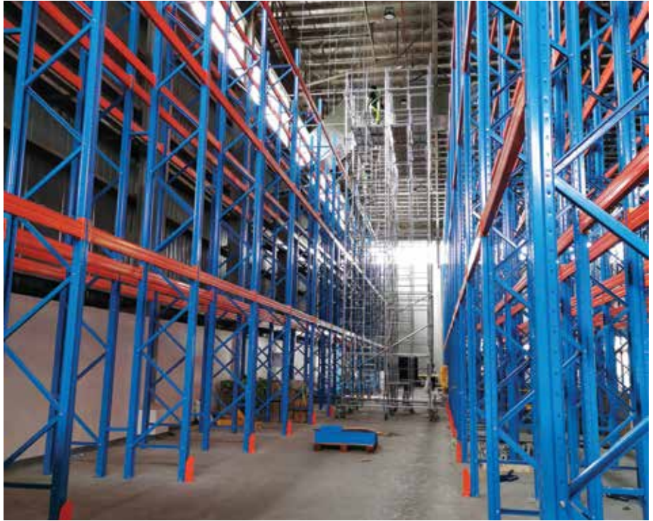
Distriphil pharmaceutical warehouse in the Philippines with 6,388 pallet positions. (Photo courtesy of Jojo Castro.)
