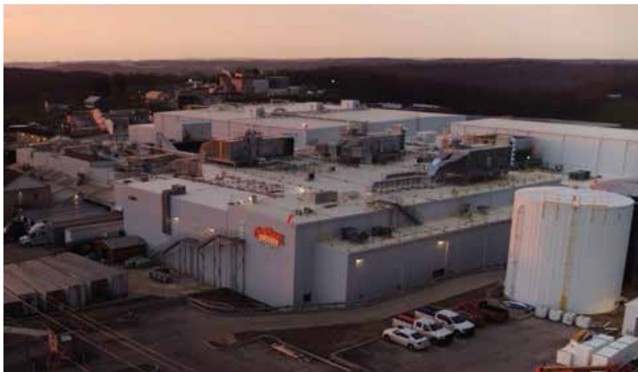
Case Farms' expanded poultry processing center in Winesburg, Ohio, built by Primus Builders, Inc. (Photo courtesy of Primus Builders, Inc.)
