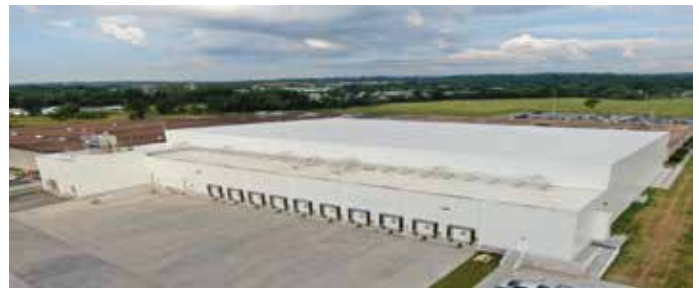
Winchester Cold Storage, Winchester, Virginia
