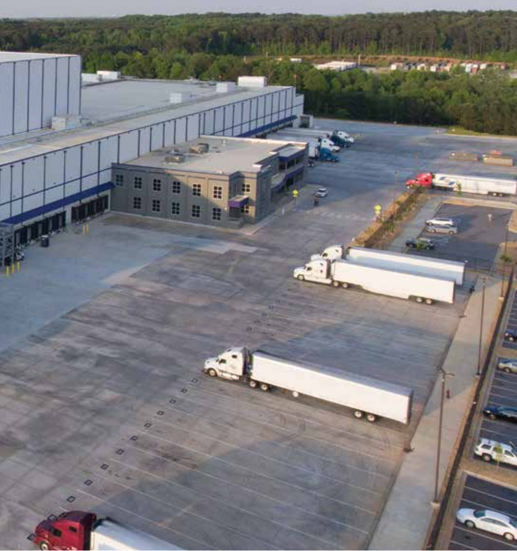
The 254,928-square-foot design-build expansion to the McDonough facility includes an ASRS cold storage and repacking facility for Dole Foods. (Photo courtesy of Fisher Construction Group.)
