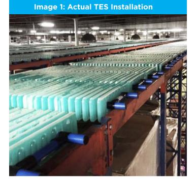
As ambient temperatures increase during peak hours of the day and the heat rejection of the condenser is less efficient, the control algorithms reduce or stage the run time of the refrigeration system and allow the fully charged TES modules (frozen PCM) to absorb the heat infiltration and maintain temperature stability inside the freezer.
