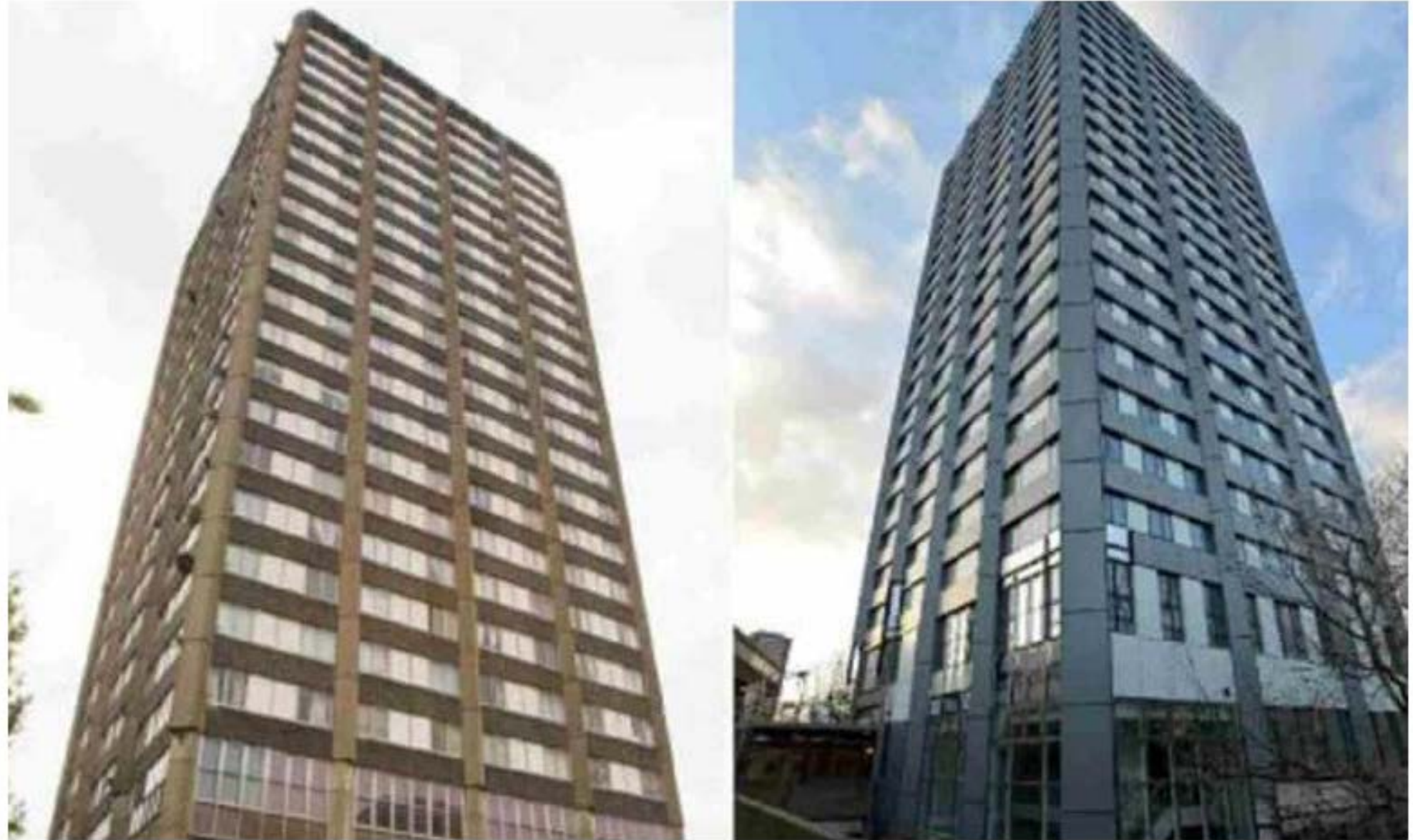
▲ Grenfell Tower before and after refurbishment work. Photograph: Grenfell Tower Inquiry/PA
